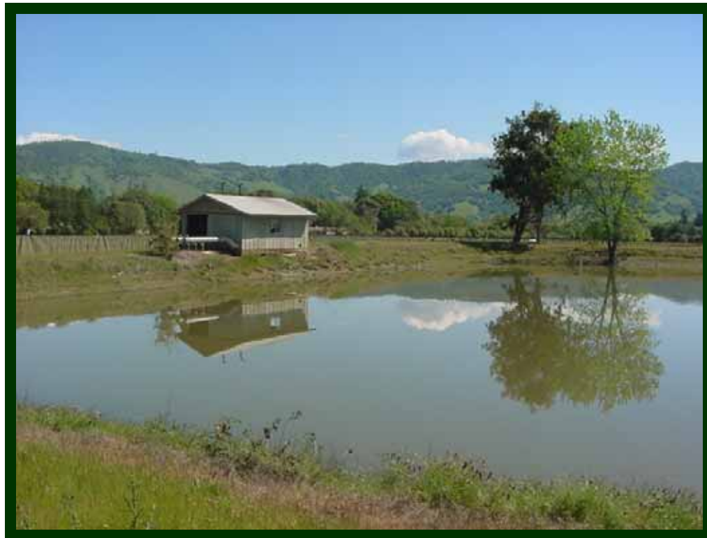
Pond & Pump House
