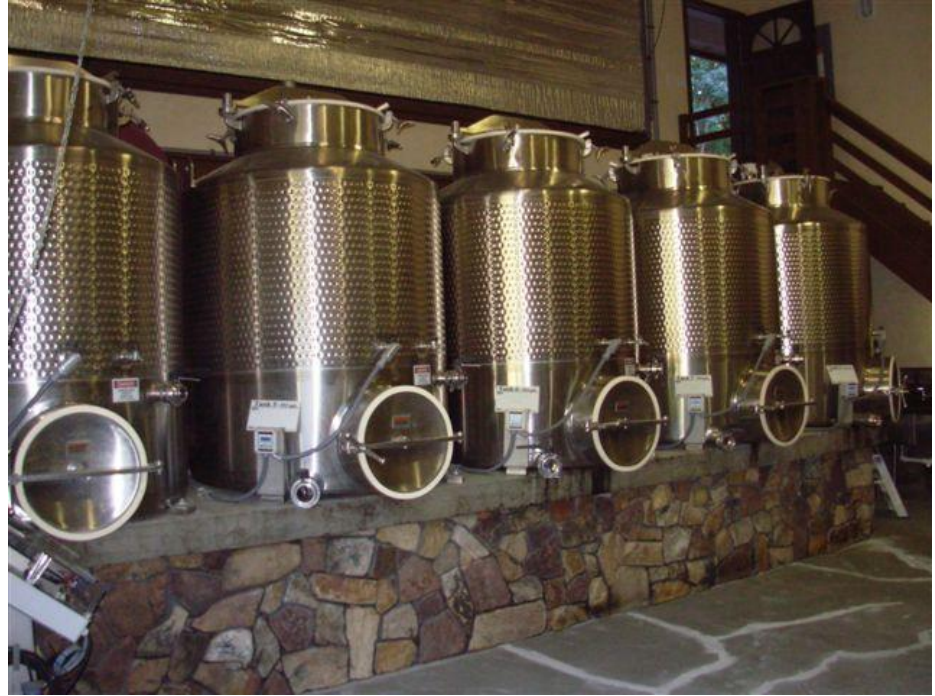
STAINLESS STEEL TANKS
